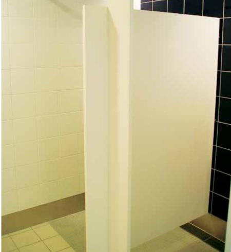
**NUVEX**<sup>®</sup> is moisture resistant and ideal for shower partitions, privacy screens and other wet area applications. The stalls are heavy duty and will not swell, splinter or rust in damp conditions. NUVEX® partitions are virtually unbreakable and chemically inert.
